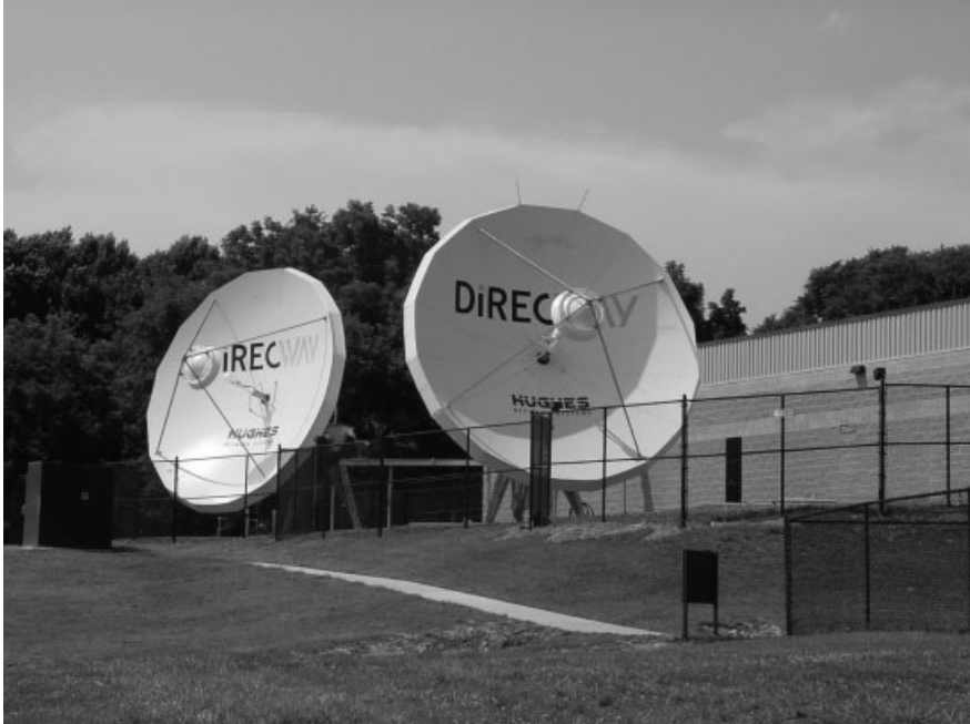
Figure 1.25 Photograph of the outdoor unit of a hub station. (Reproduced by permission of Hughes Network Systems, Inc.)
