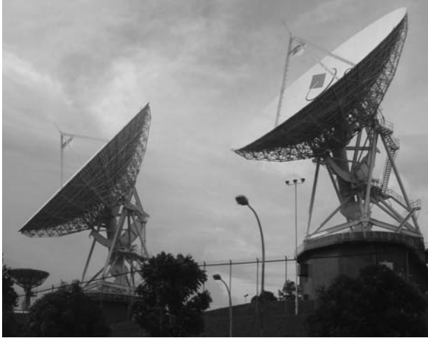
Figure 8.51 Bukit Timah Satellite Earth Station (Author: mailer_diablo )
